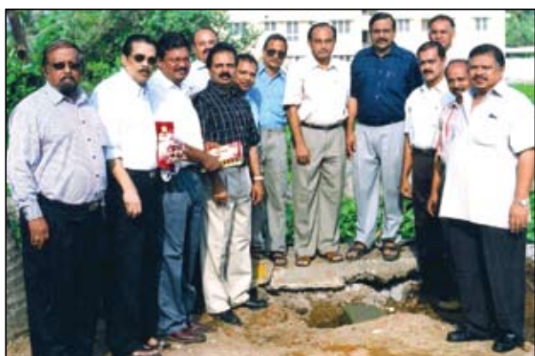
29th March 2006 - The foundation stone being laid by Dr. S. S. Kamath and Dr. E. Varghese Mathew to construct a bridge across canal in front of IMA Site.
