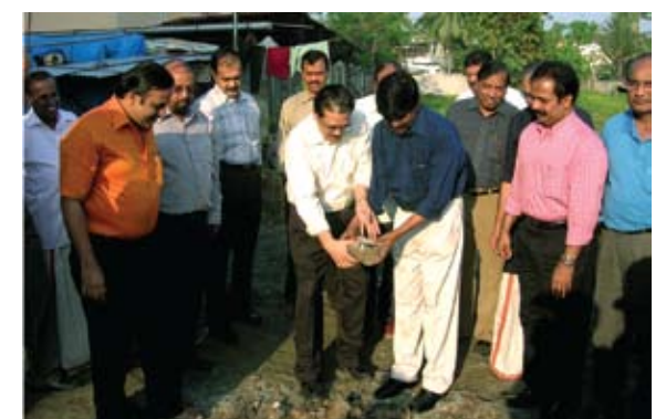
5th March 2008 - Bhoomi Pooja for 2nd block. Foundation stone laid by Dr. V.P. Kuriyipe & Dr. N.S.D. Raju
